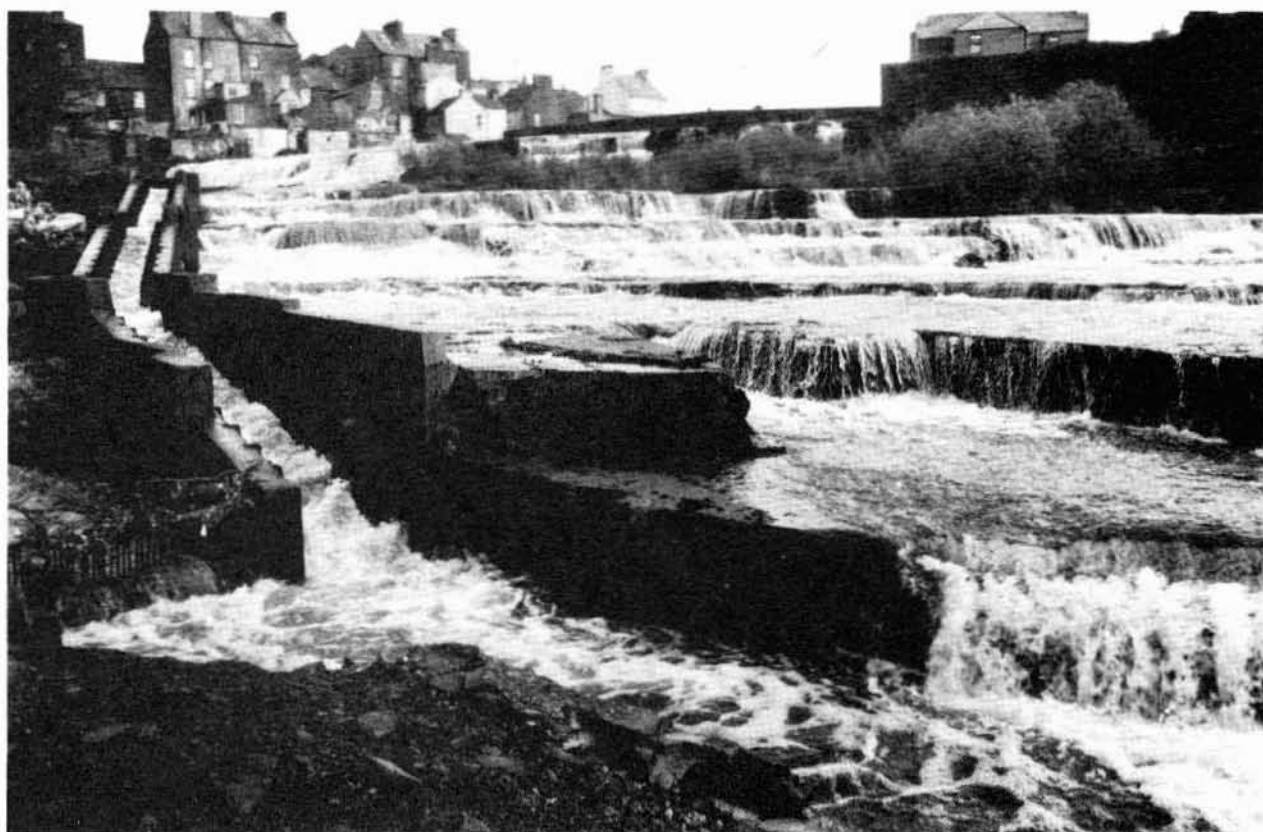
Figure 19 A view up part of the extensive Denil fish pass complex at Ennistymon on the River Inagh in the Republic of Ireland.
