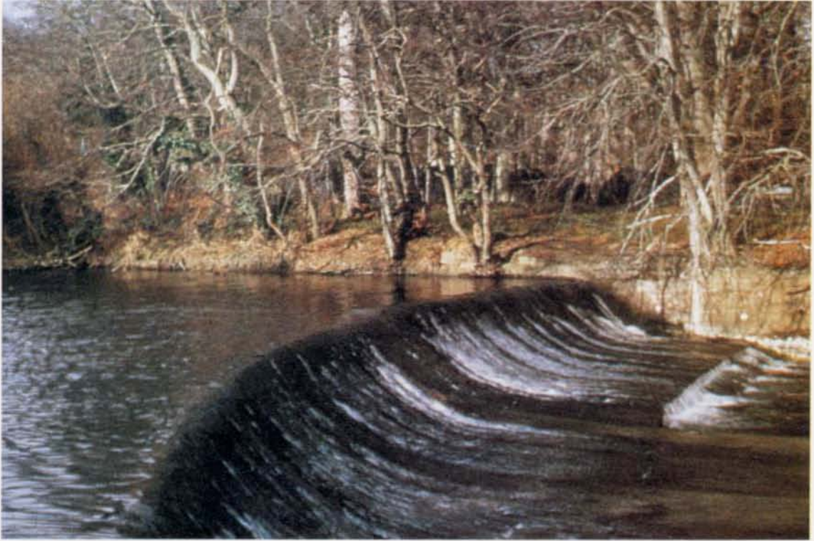
3 - Warkworth Dam, River Coquet (UK): traversa insuperabile a causa del profilo concavo
